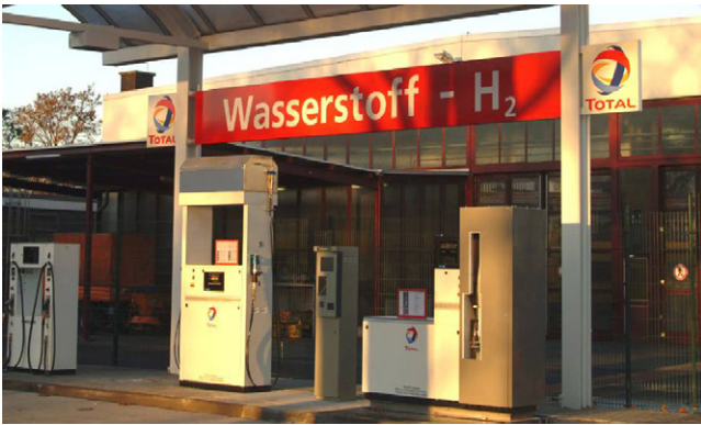
Fig. 2. TOTAL hydrogen-filling station at Heerstraße, Berlin.
