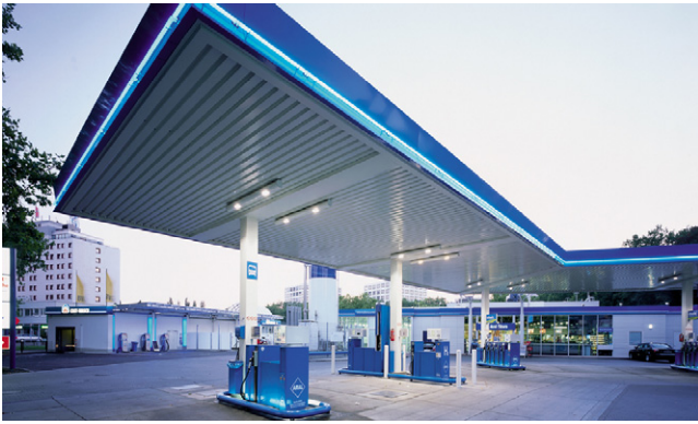
Fig. 1. Aral/BP hydrogen-filling station at Messedamm, Berlin.
